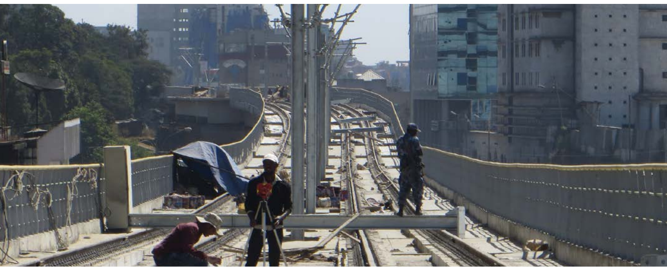
Light rail construction in Addis Abeba.
